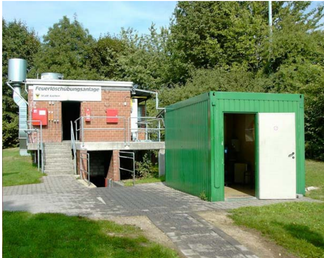
Hot fire training lab
